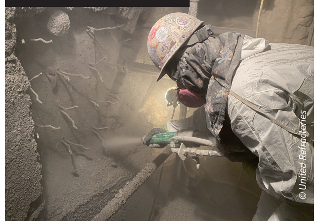
Figure 1: low dust emissions in a lower cyclone cement-free gunite repair
