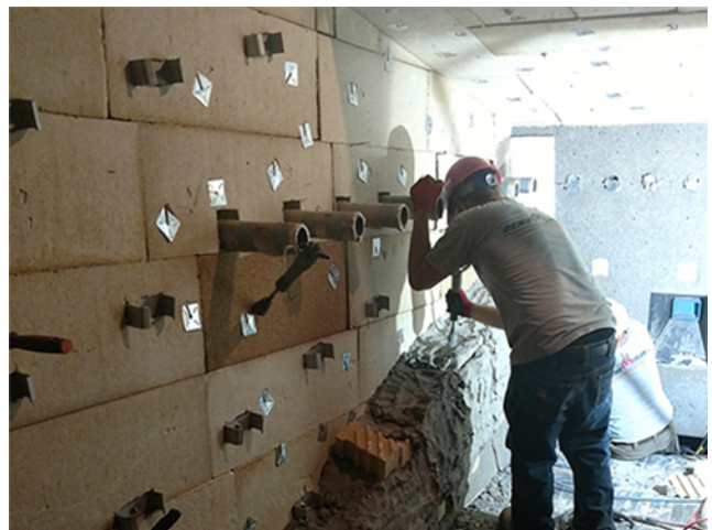
Figure 4. Ramming plastic on a side wall.
