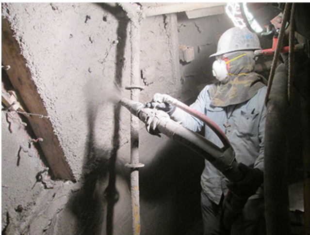
Figure 2. Shotcreting onto a side wall.
