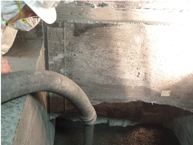
Figure 1. Pump mix being installed into a form.
