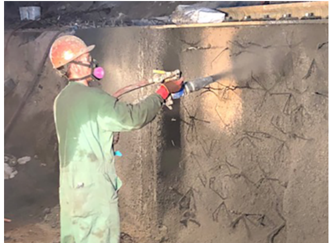
Figure 3. Gunning onto a side wall.
