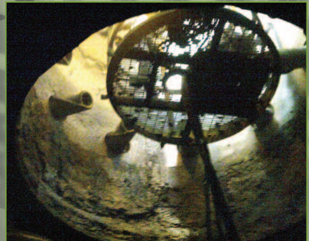
The cupola veneering process takes place in tight quarters, making the excellent gunnability and "sticky nature" of the UNI-GUN low cement mixes critical features for success.
