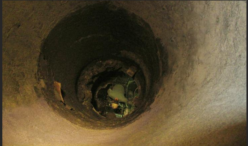
LEFT: Prior to installation of the shotcrete, metal anchors were applied in the upper stack.
