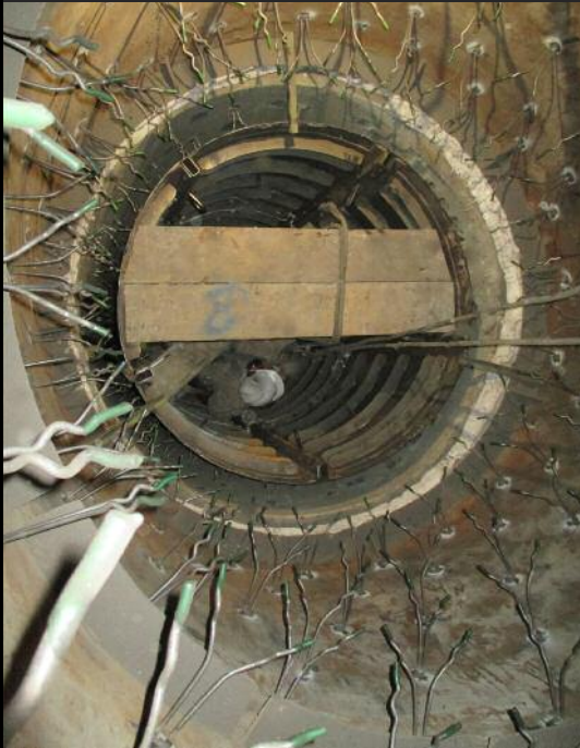
LEFT: Prior to installation of the shotcrete, metal anchors were applied in the upper stack.
